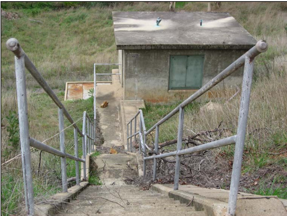
Plate 14: Bailey valve hut at Oberon Dam showing access steps. View is from west.
