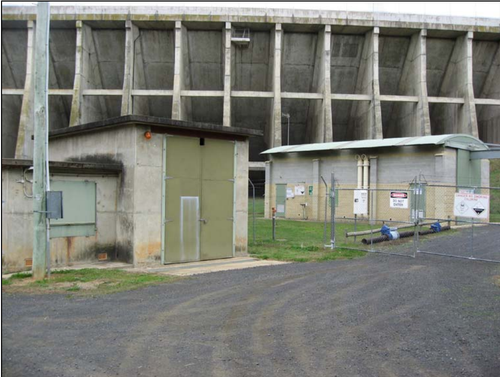
Plate 15: Disused chlorinator hut (left) and new chlorinator hut (right) at Oberon Dam (background). View is from north-west.
