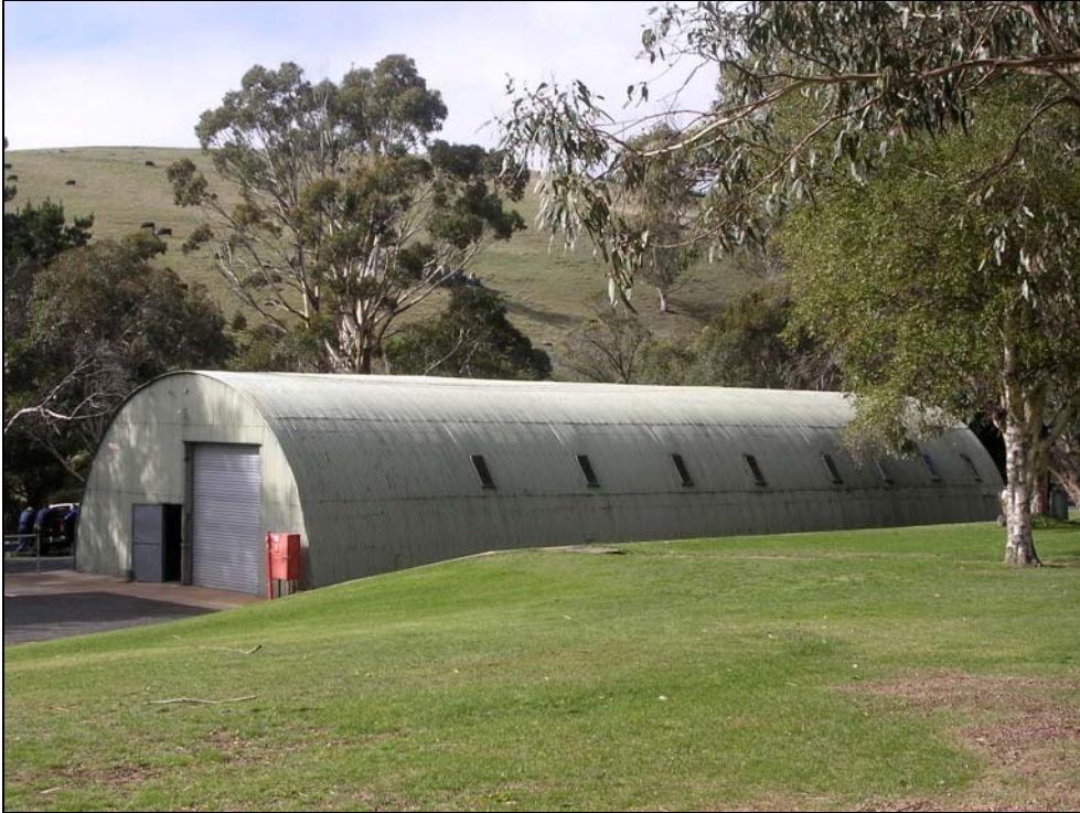
Plate 9: Pre-fabricated semi-cylindrical hut/workshop at Oberon Dam. View is from west.
