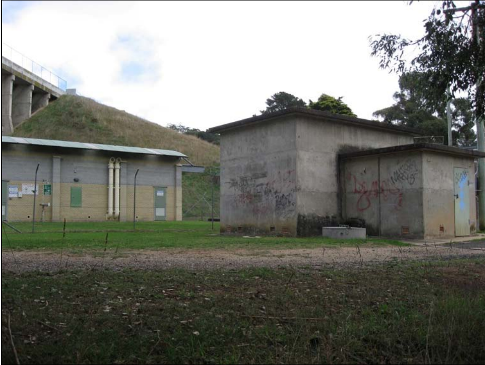
Plate 17: Disused chlorinator hut at Oberon Dam, showing wall graffiti. View is from south.
