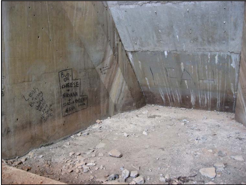
Plate 3: Oberon Dam, showing detail of graffiti within buttress area. View is from north.
