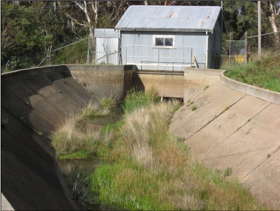
Plate 19: Break pressure tank at Duckmaloi showing concrete channel and eastern end valve hut. Note vegetation in channel. View is from centre of break pressure tank.
