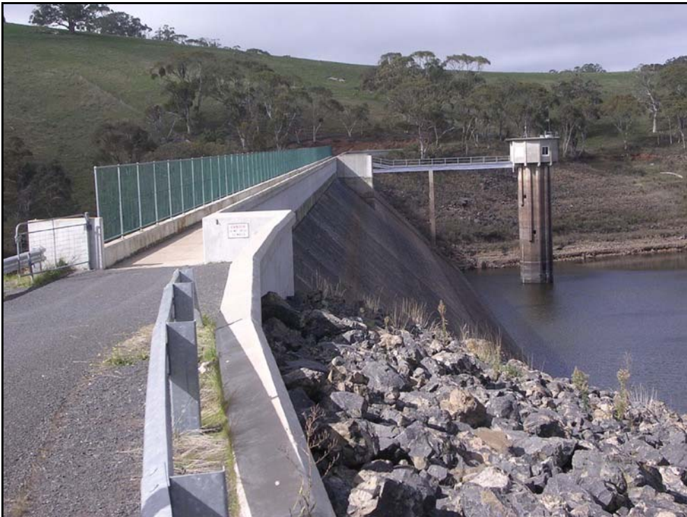
Plate 2: Oberon Dam, showing parapet, safety fencing and control tower. View is from west.
