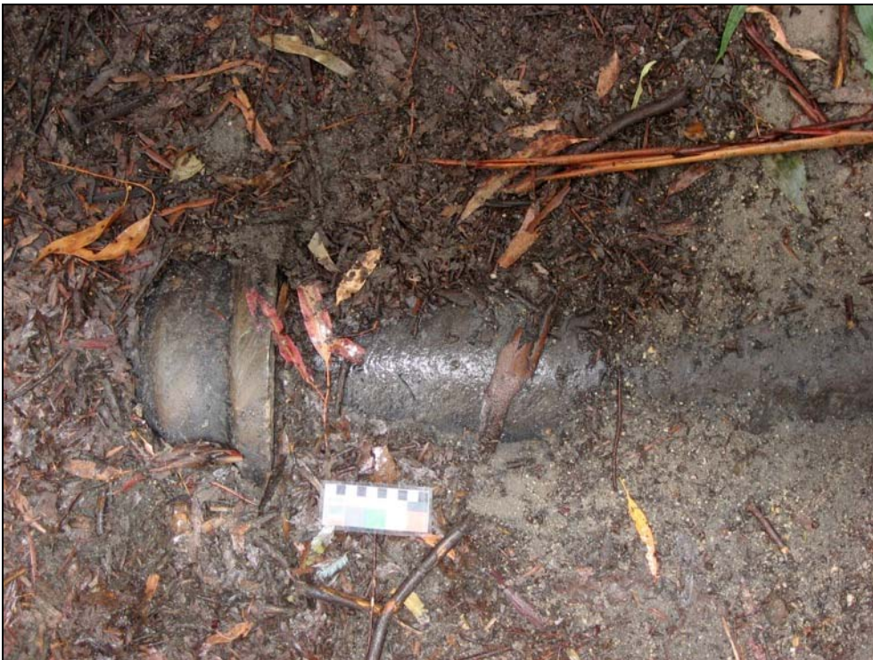
Plate 35: FRWS pipeline in the vicinity of Baal Bone Gap. Detail of exposed pipe.
