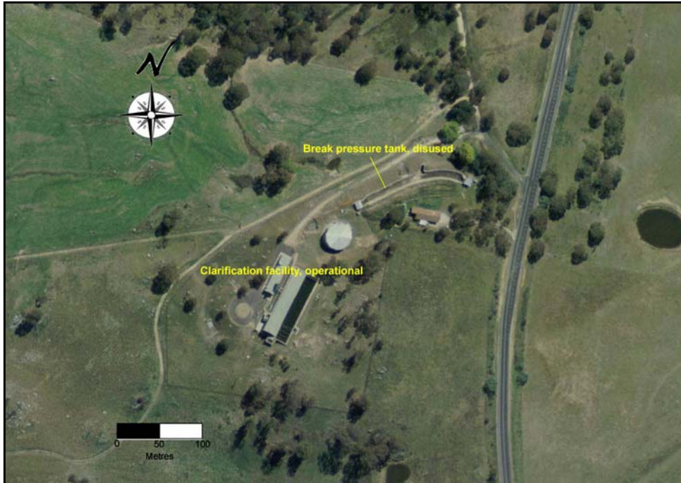
Figure 5: Duckmaloi water treatment plant and break pressure tank (Source: Department of Lands)
