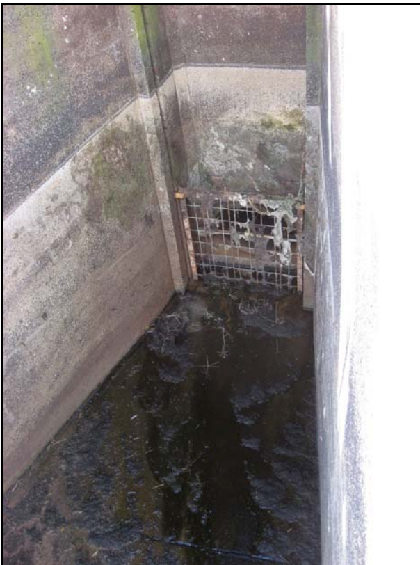
Plate 20: Break pressure tank at Duckmaloi showing central screening chamber outlet.
