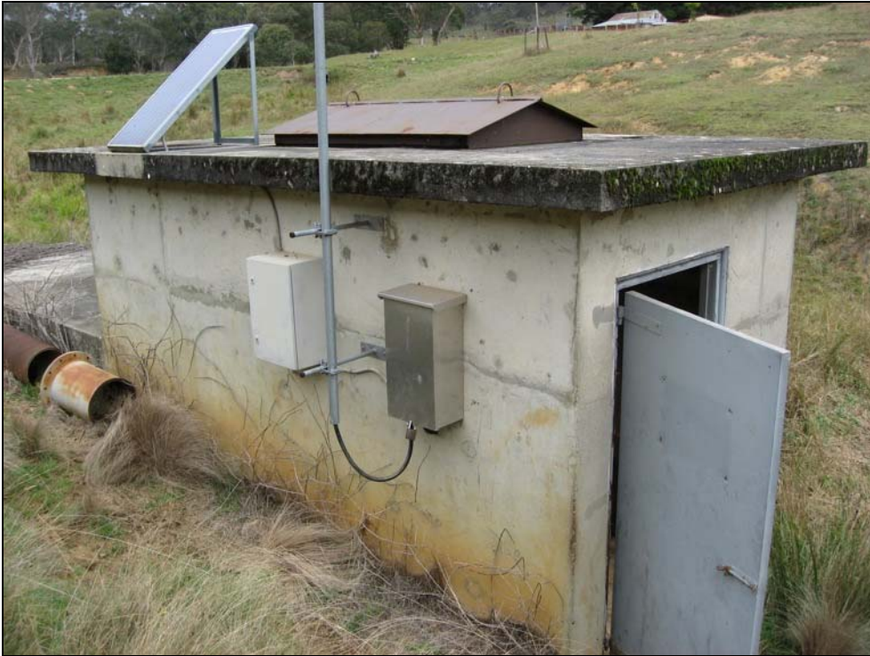
Plate 21: Hampton Tunnel inlet chamber. View is from north-west.
