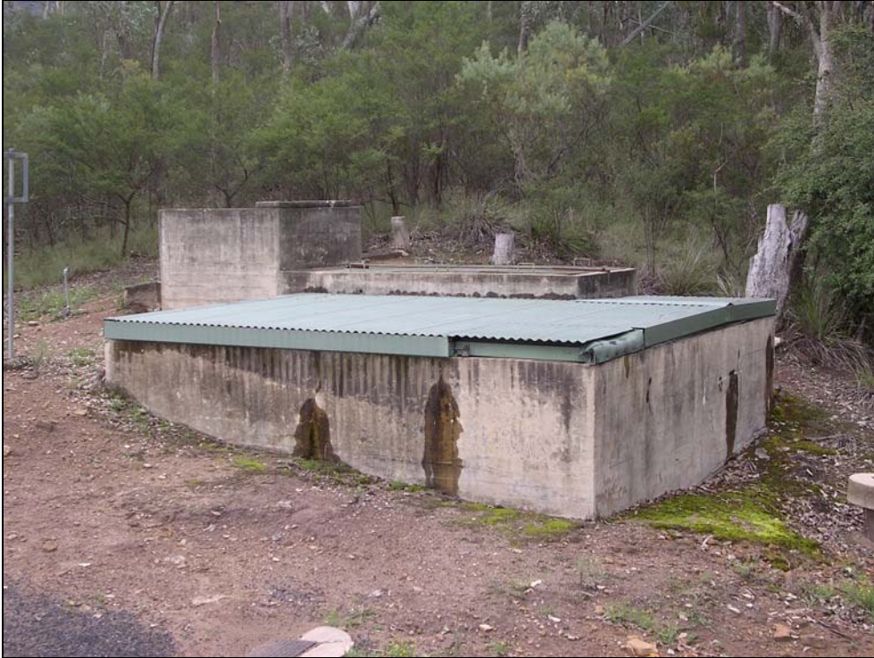
Plate 32: Glen Davis pup tank. View is from west.
