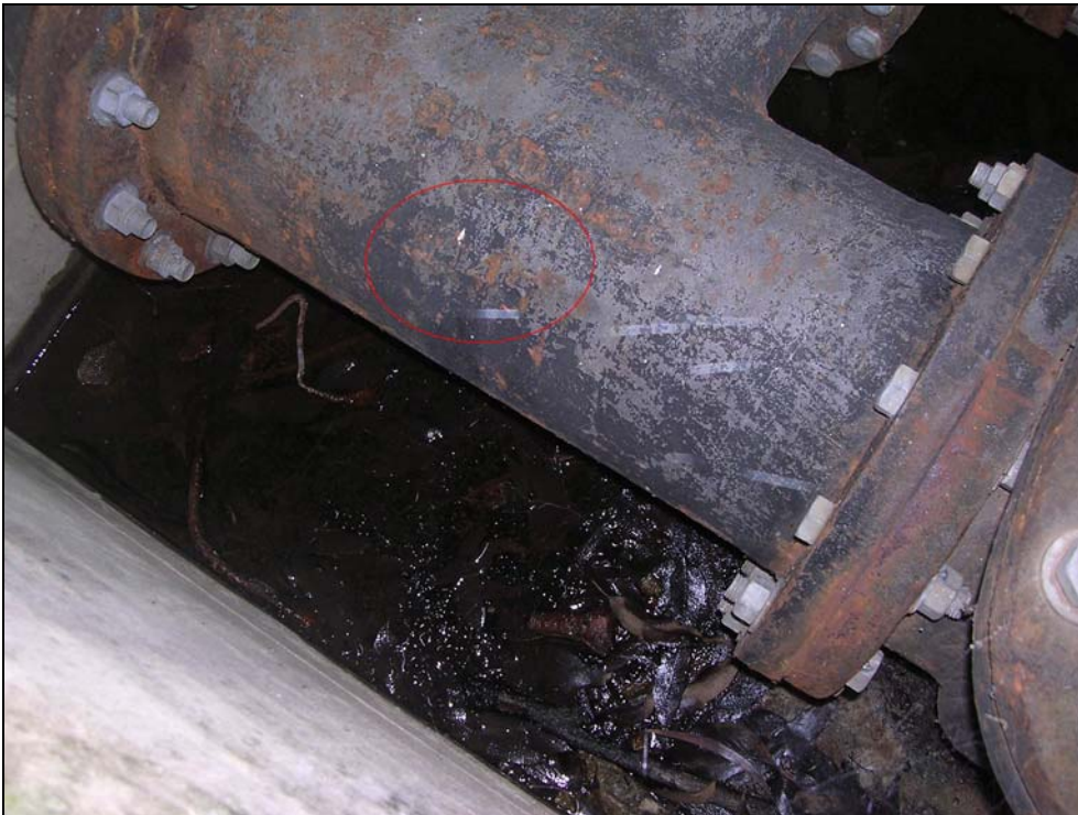
Plate 33: Glen Davis pup tank, detail of date stamp on internal pipe reading 1945.
