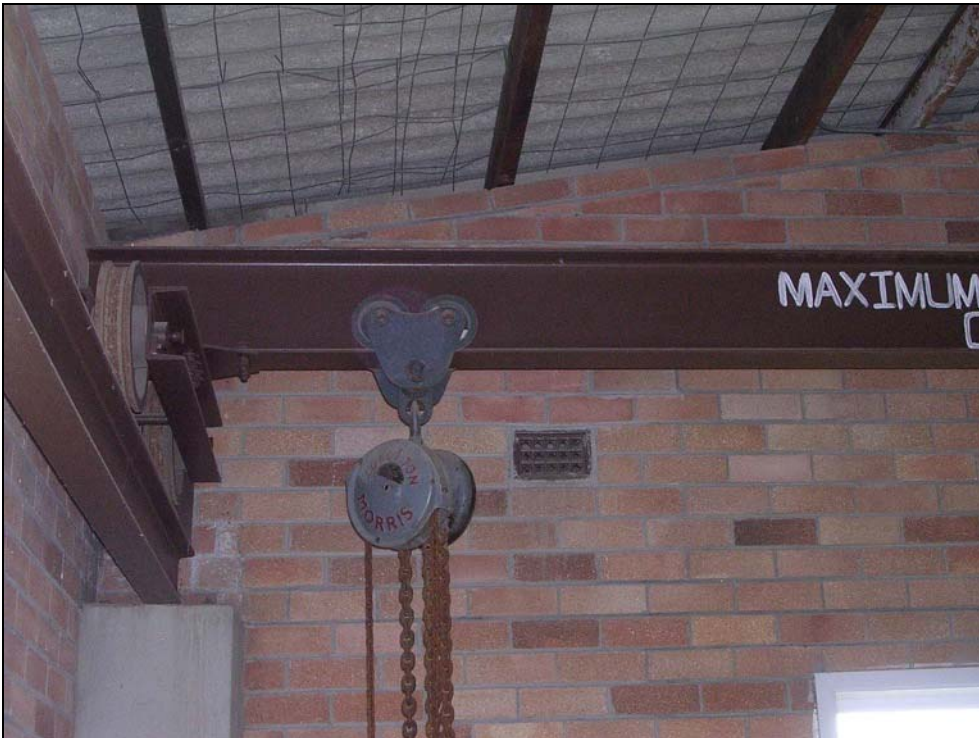
Plate 27: Wallerawang Pumping Station, interior, showing detail of original pulley and chain components.
