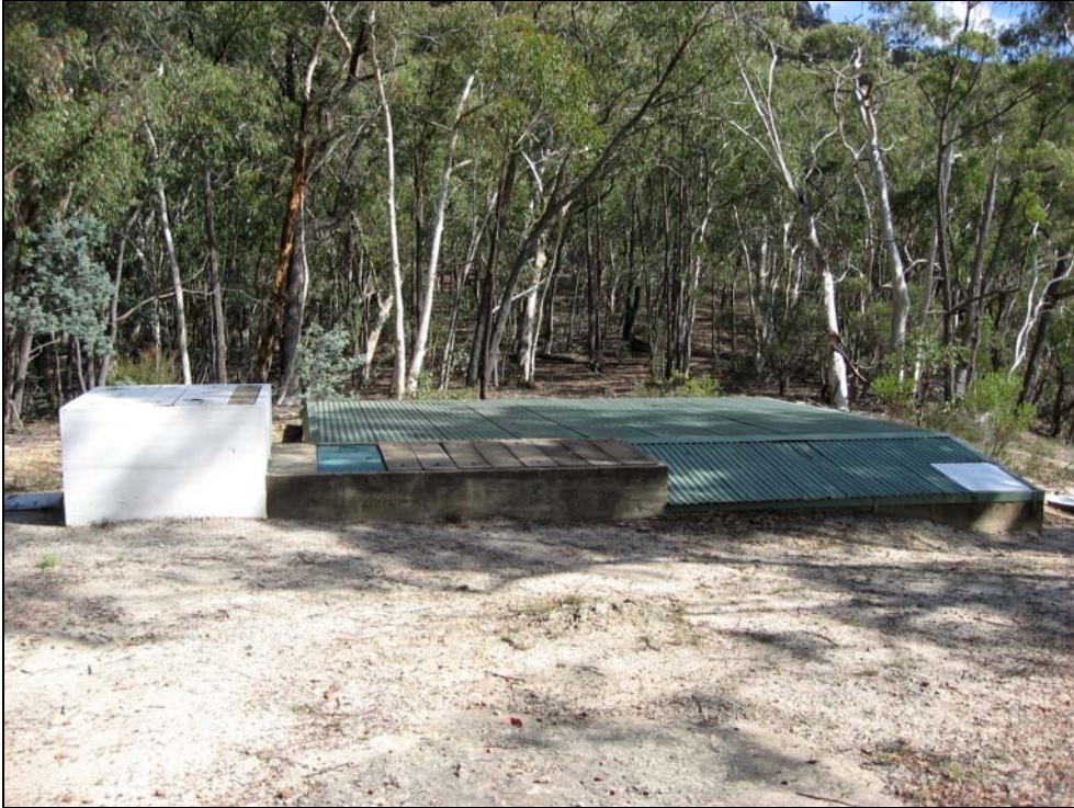
Plate 36: Break Pressure Tank 1 at Baal Bone Gap, showing the new fabric of the superstructure.
