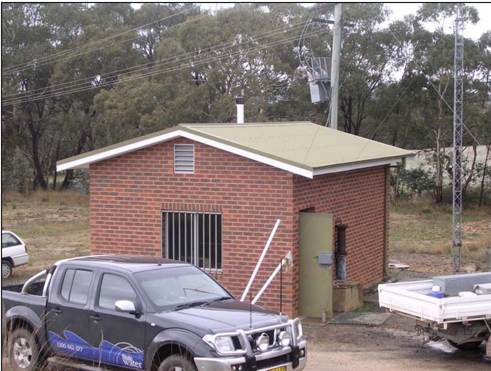
Plate 25: Rydal Dam, showing valve hut and vehicle car park. Current valve hut fabric encases original valve hut fabric.
