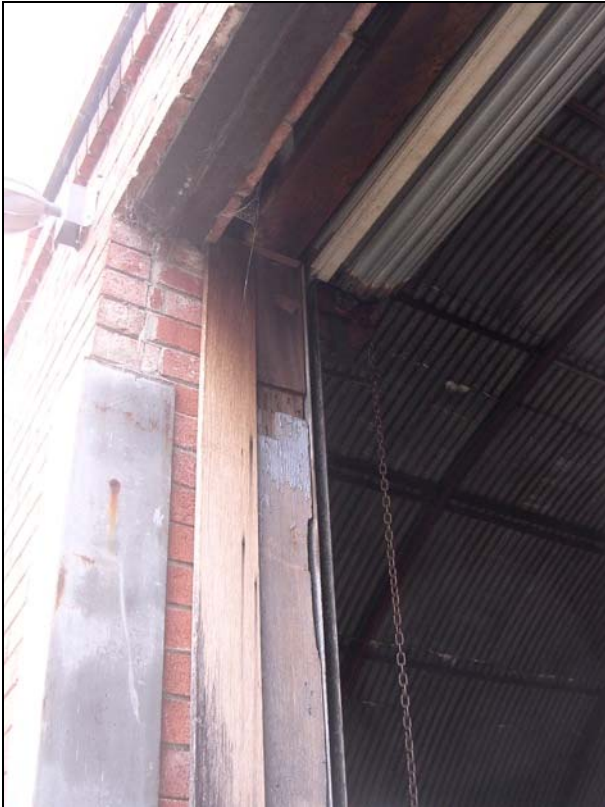
Plate 30: Wallerawang Depot, pre-fabricated semi-cylindrical hut/workshop, showing original door frame and brackets at rear of building.
