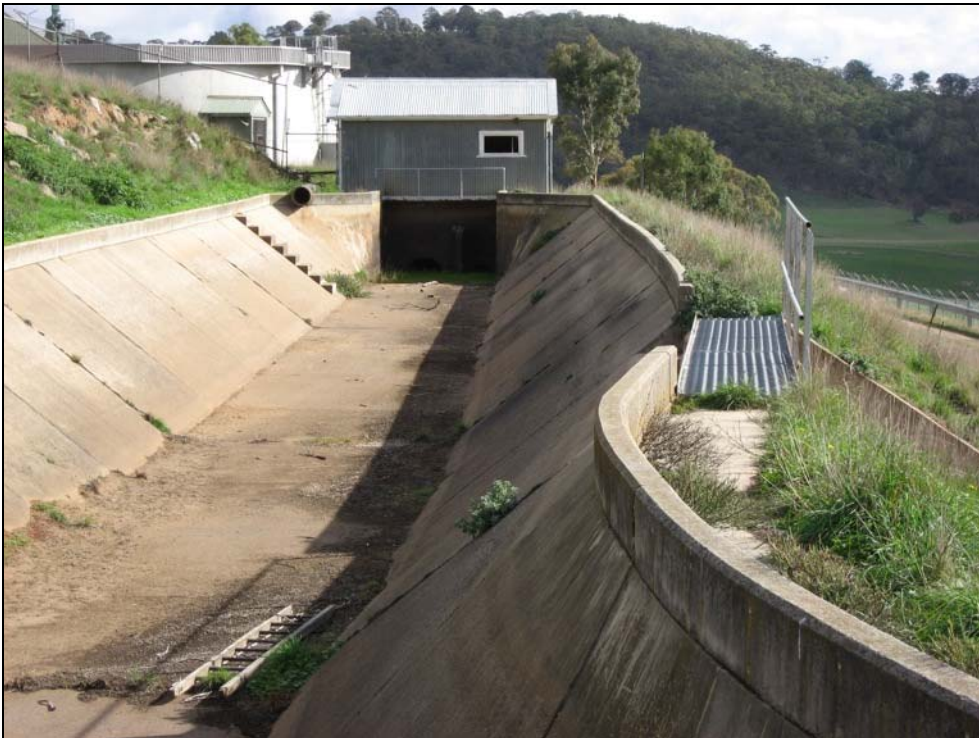
Plate 18: Break pressure tank at Duckmaloi showing concrete channel and western end valve hut. View is from centre of break pressure tank.
