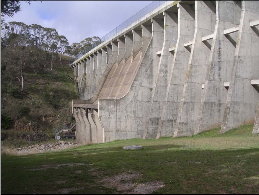
Plate 1: Oberon Dam, showing dam wall buttresses and ski-jump spillway. View is from west.
