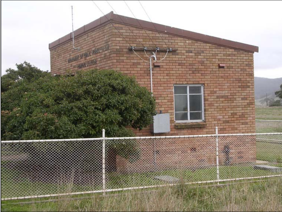
Plate 26: Wallerawang Pumping Station.
