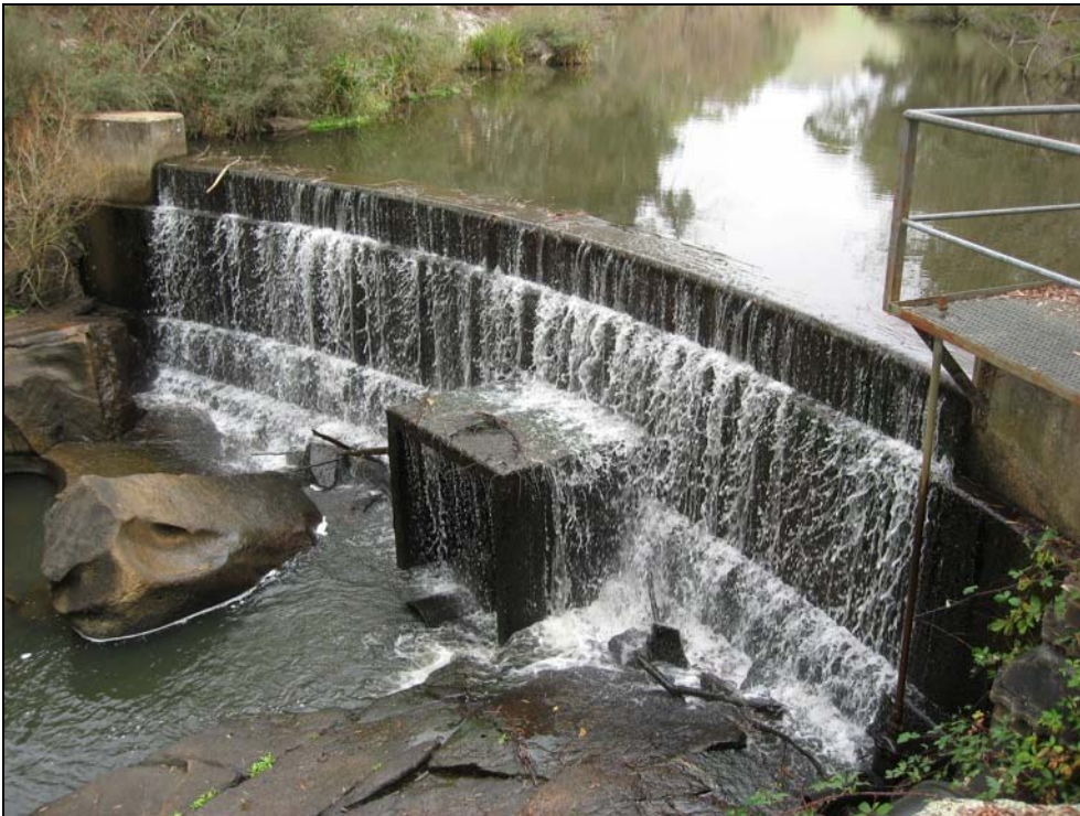
Plate 23: Duckmaloi Weir showing intact dam wall.
