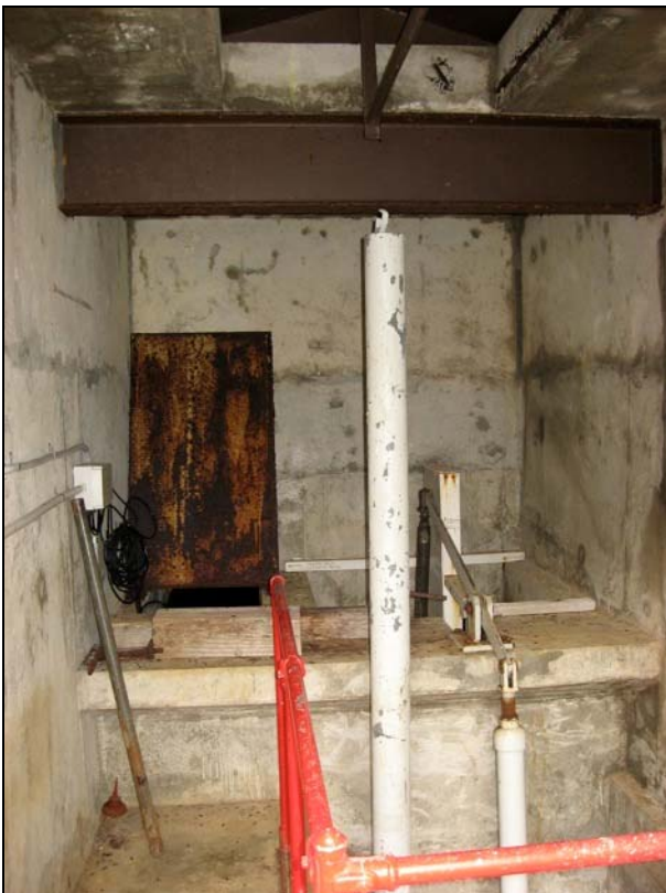
Plate 22: Hampton Tunnel inlet chamber. Interior.
