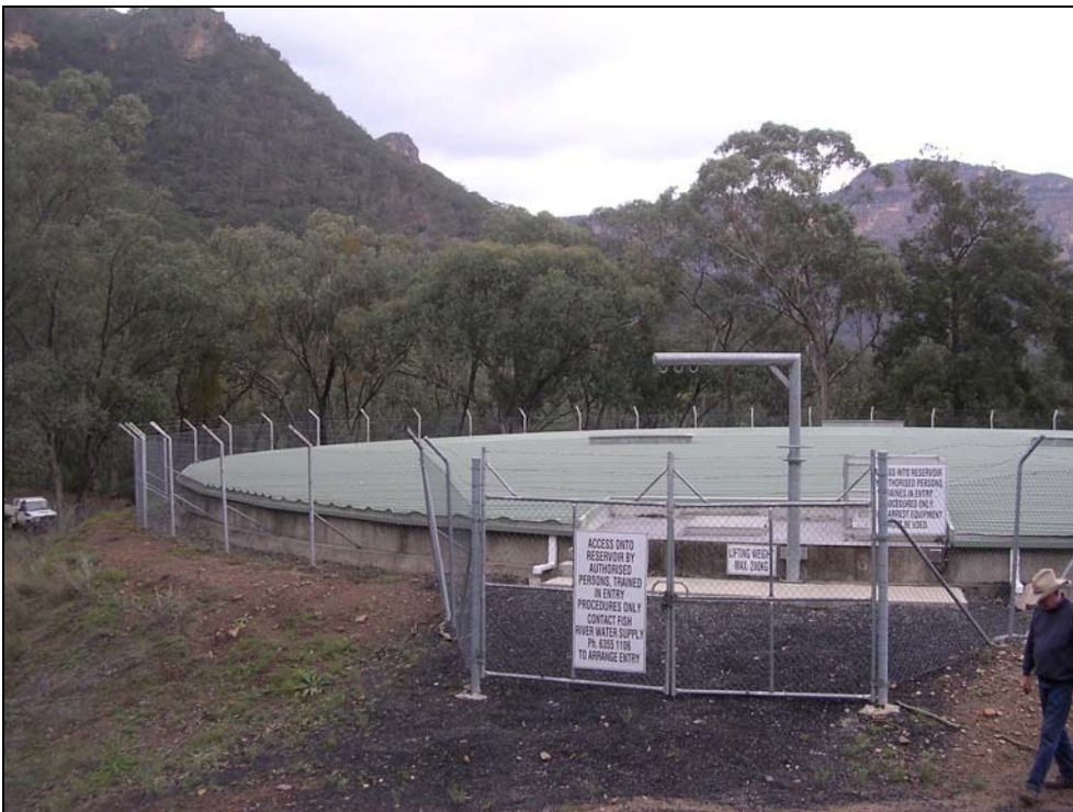
Plate 31: Glen Davis reservoir tank. View from east.
