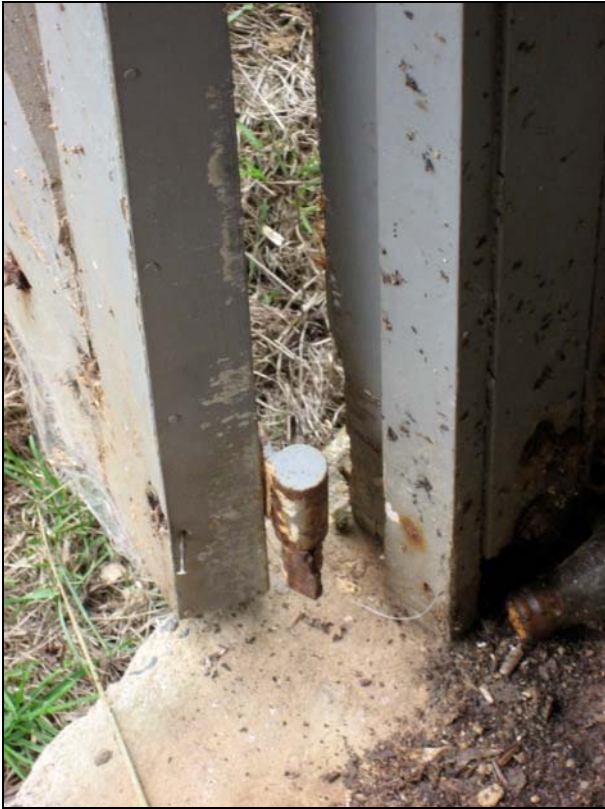
Plate 23: Hampton Tunnel inlet chamber. Detail of broken hinge.
