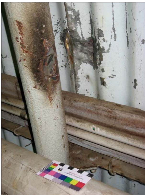
Plate 12: Pre-fabricated semi-cylindrical hut/workshop at Oberon Dam. Detail showing minor damage to lower part of rib.
