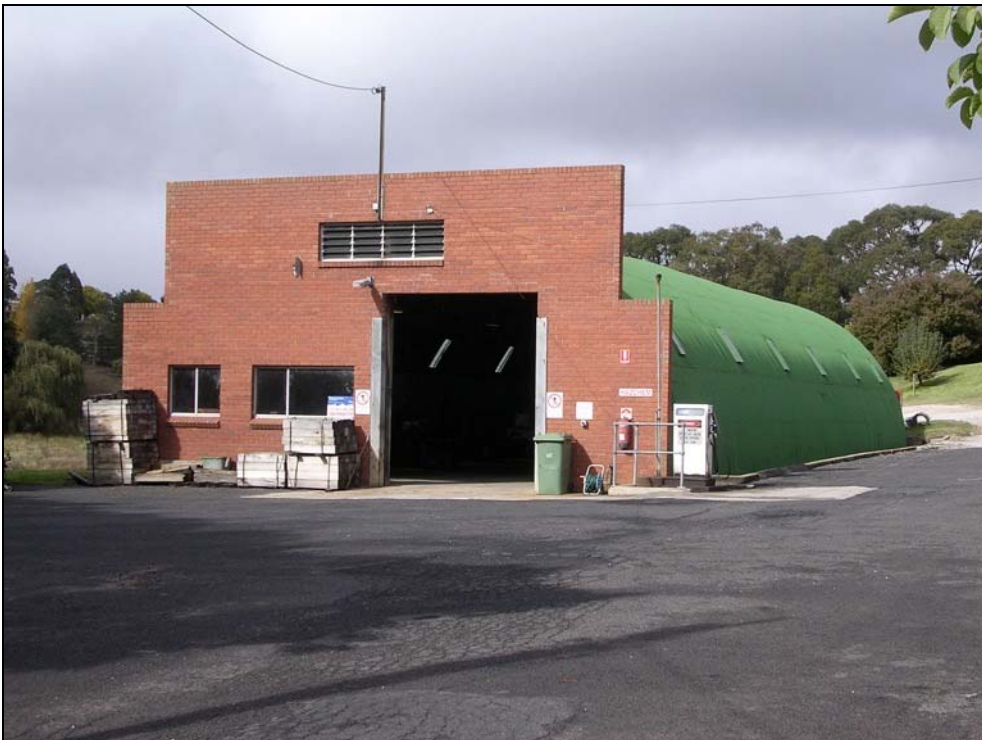
Plate 29: Wallerawang Depot, pre-fabricated semi-cylindrical hut/workshop, showing new façade. View is from north.
