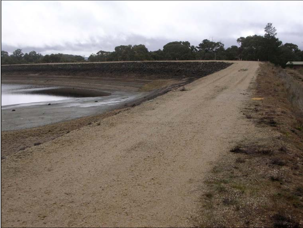
Plate 24: Rydal Dam, showing recently rebuilt dam wall. Chlorinator hut is visible in top-right of photograph. Valve hut is situated out-of-shot to the right of the photograph.
